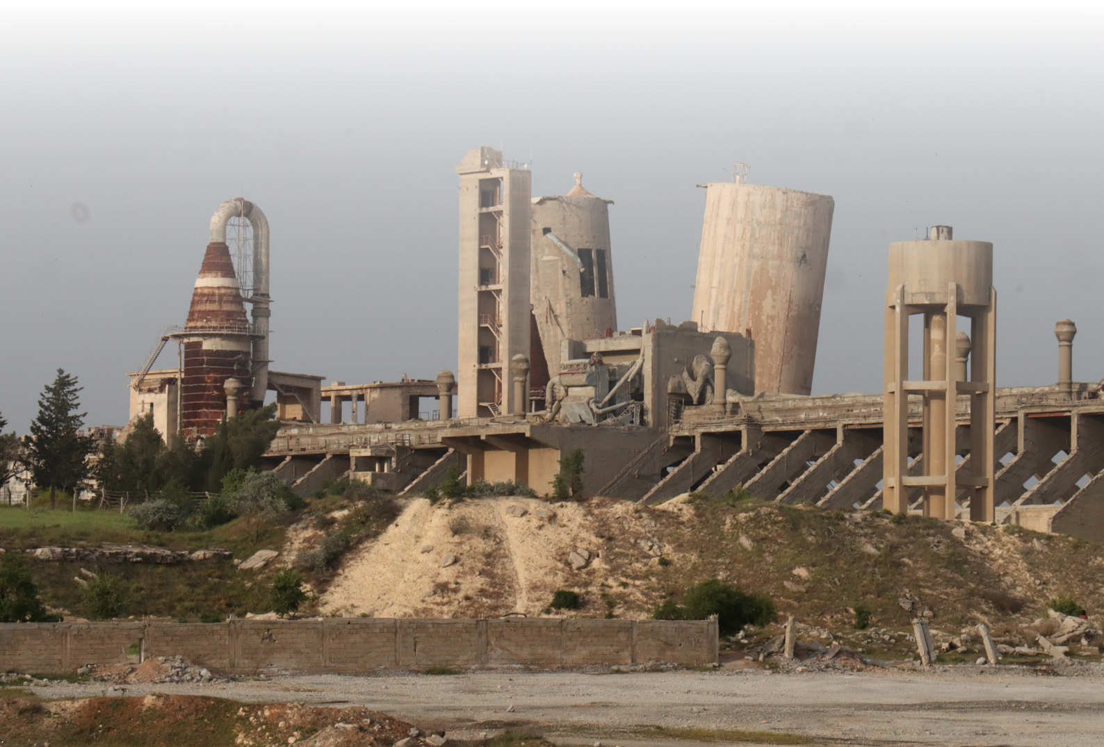
Destroyed cement factory near Ma'arat al-Muslimiya village, November 2022
