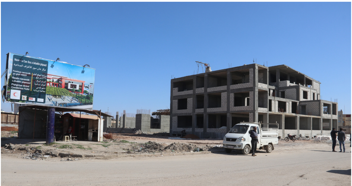
THE NEW HEALTH CENTER IN CONSTRUCTION, FEBRUARY 2021
